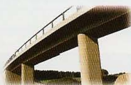
a concrete bridge
